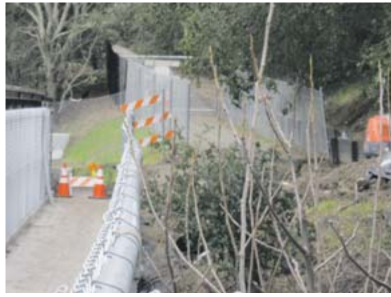
Canyon Bridge pedestrian access closed Photo Vera Kochan
